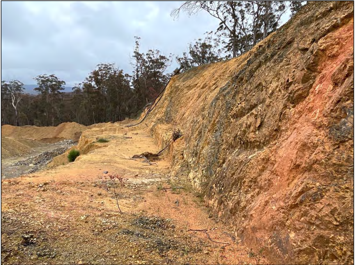
Figure 8: Looking north along the existing cut batter and bench in the eastern part of the quarry (typically very low strength siltstone exposed).
